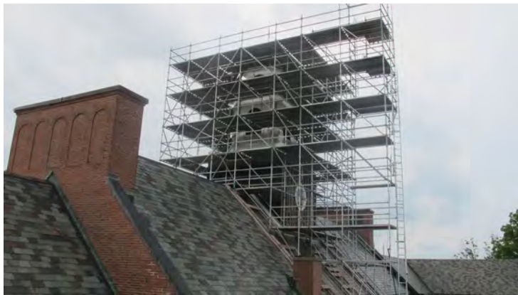
Roof view of cupola facade restoration at Mexico High.
