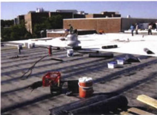
Eastern Suffolk B.O.C.E.S.- Roof Replacment
