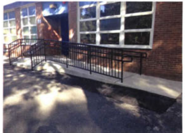
Port Washington UFSD – ADA Upgrades
