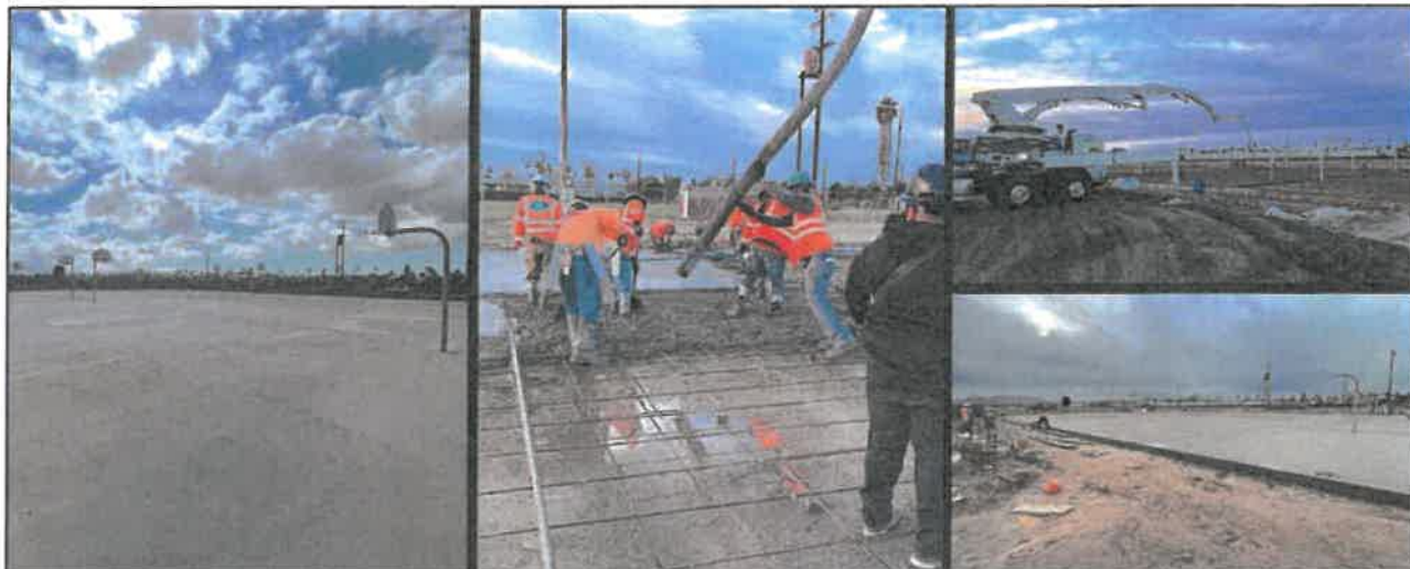
New Basketball Courts Placing of the concrete and basketball posts
