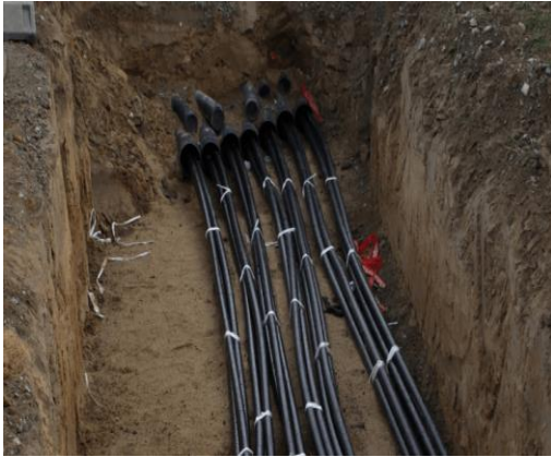
Olga Reed Elementary School Underground Electrical Project
