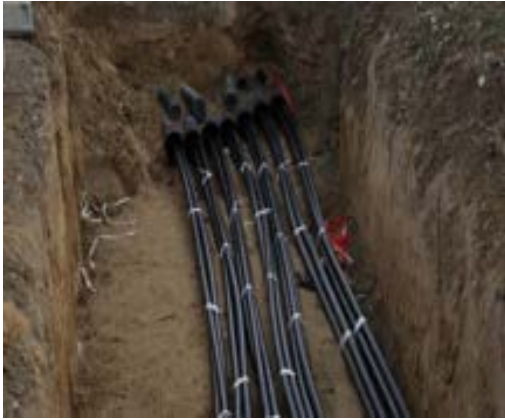
Olga Reed Elementary School Underground Electrical Project
