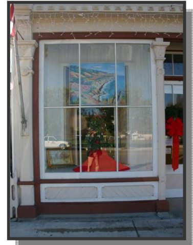
Fig. 4.9: Classic wood detailing for storefront with trim, multiple glass panes, and ornamented pilasters.
