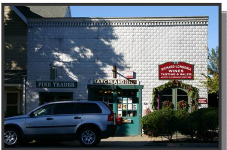
Fig. 4.8: Metal clad frame structure with material stamped to represent stone.
