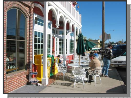
Fig. 3.3: Porch overhang maintains zero setback but covers widened sidewalk for tables and entry area.
