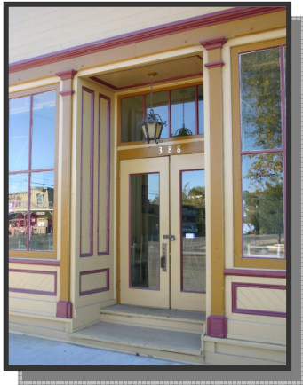
Fig. 5.1: Recessed entry with detailed painted wood trim at sides give character at the pedestrian level.
