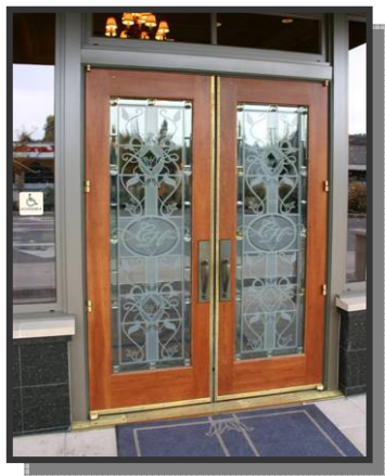
Fig. 5.2: Wood door with elaborate sand-blasted glazing and tile at floor of entry.
