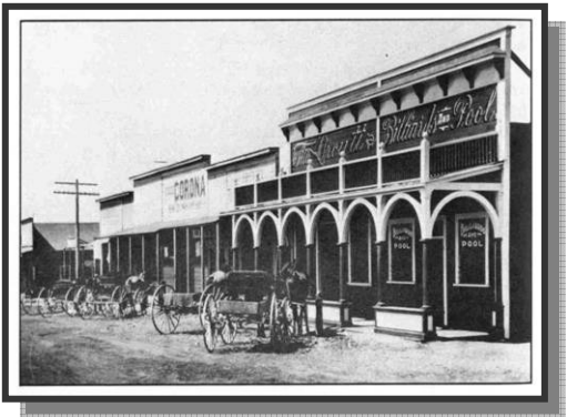
Fig. 2.5: Street scene from Old Town Orcutt along Clark Avenue. Note continuity of sidewalk, pedimented falsefront to the left and even diagonal parking.
