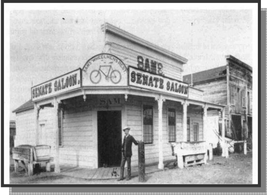
Fig. 2.4: A wood corner structure with a corner entry demonstrating a corniced falsefront, detailed posts with ornate capitals, and shadowed lettering on signs.
