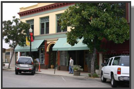
Fig. 4.7: Masonry and trowelled concrete stucco structure with detailed cornice.
