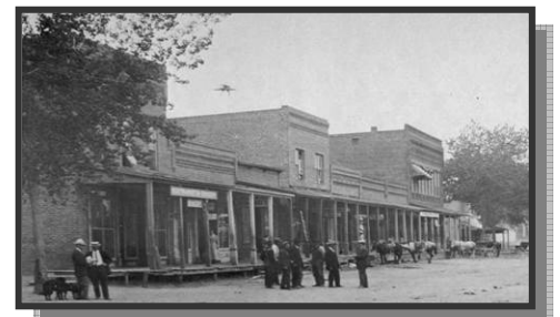
Fig. 2.3: A western street scene showing a mixture of wood and masonry structures of one and two stories but with a continuous covered boardwalk.
