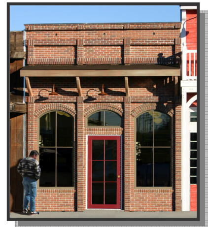
Fig. 2.2: Building replicates a classically proportioned masonry structure with three bays and a center entry. Note projected wood awning and gooseneck light fixtures.
