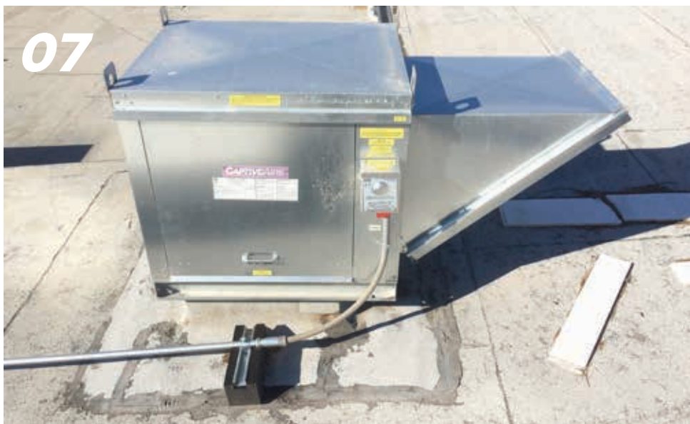
Figure 6: Exhaust Fan
