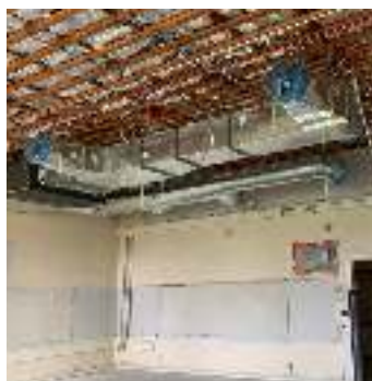
Installation of air conditioning equipment in a classroom at Madison Elementary
