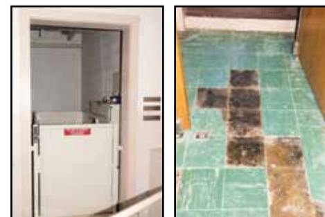
A wheelchair lift was added to make the building ADA compliant.
