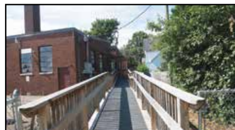
To make the backdoor exit to the playground ADA compliant, a 48' ramp had to be built to meet the needs of children unable to use the steps.
