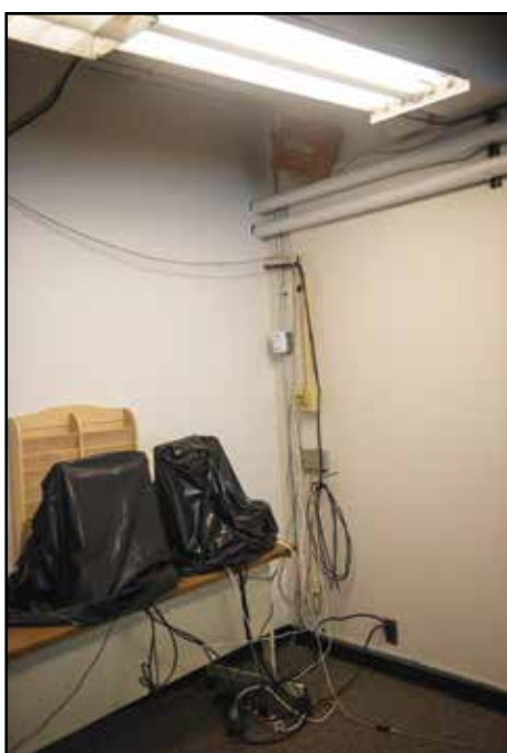
Clearmount was built before architects knew the need for multiple power outlets because of the importance of technology.
