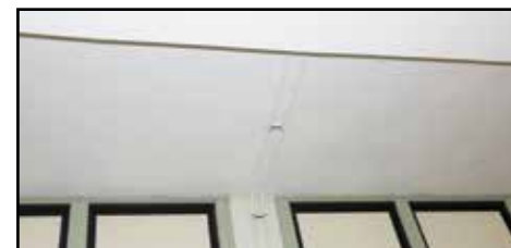
The heating pipes are run on the inside of the gymnasium.
