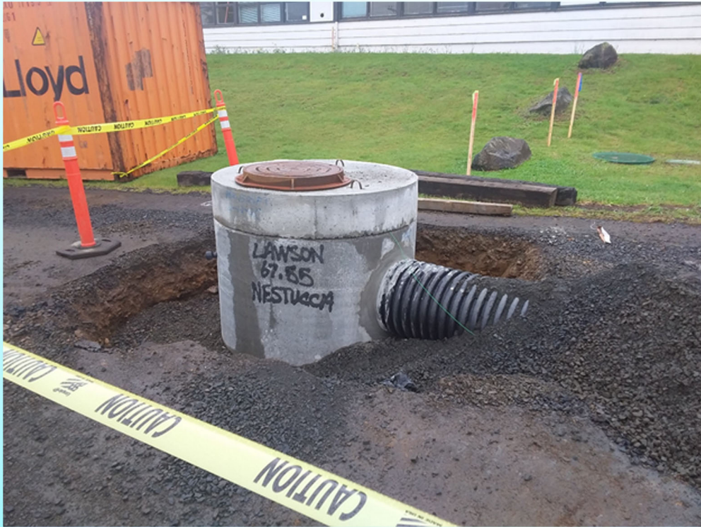
Storm line work goes in in front of school
