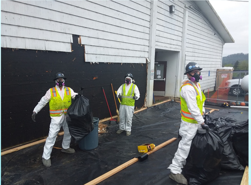
Siding demolition under way
