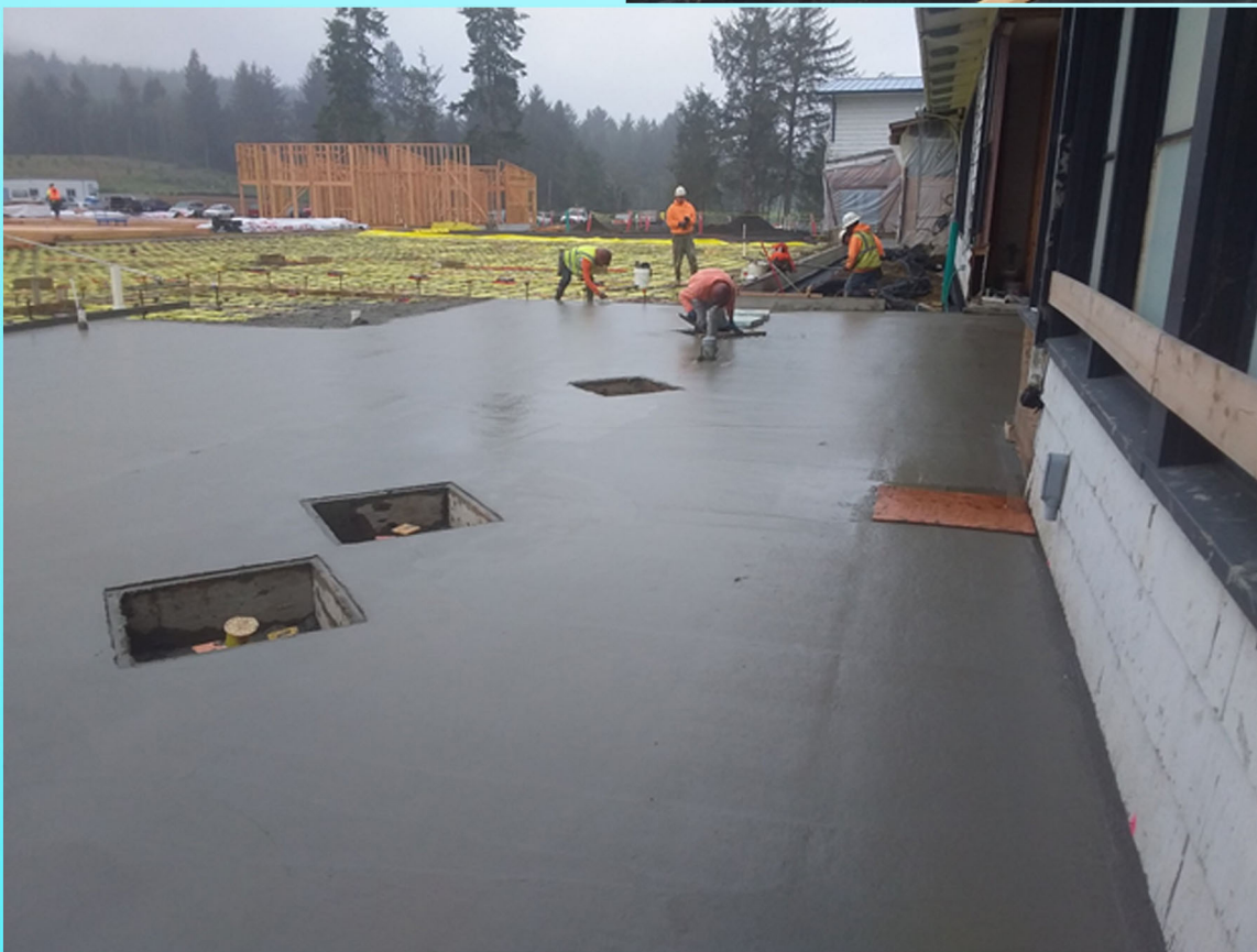
Pouring concrete that will tie in with existing school building
