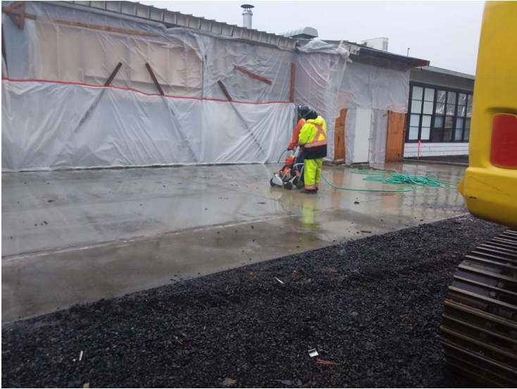
Saw cutting cafeteria slab for removal
