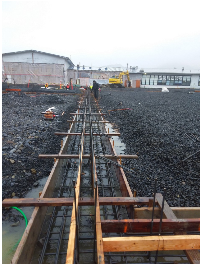
some steel tied in gym spread footing
