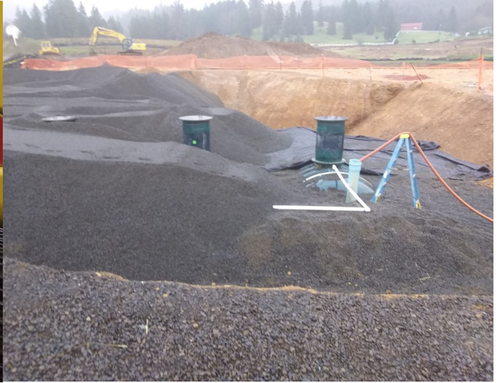
Xerxes tanks are getting some cover
