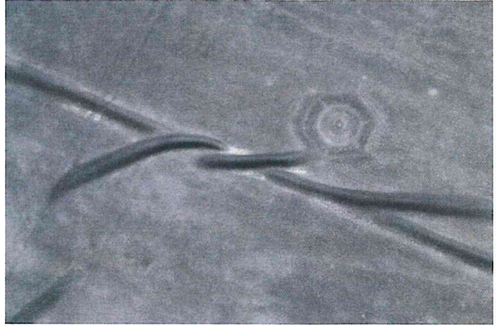
Wrinkles in EPDM will telegraph through the AlphaGuard system. It is necessary to make these repairs before applying AlphaGuard.
