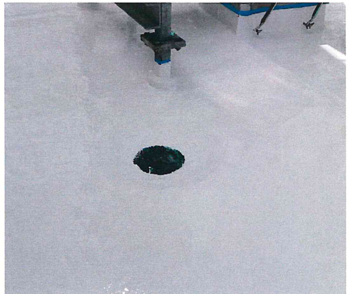
Completed drain detail.
