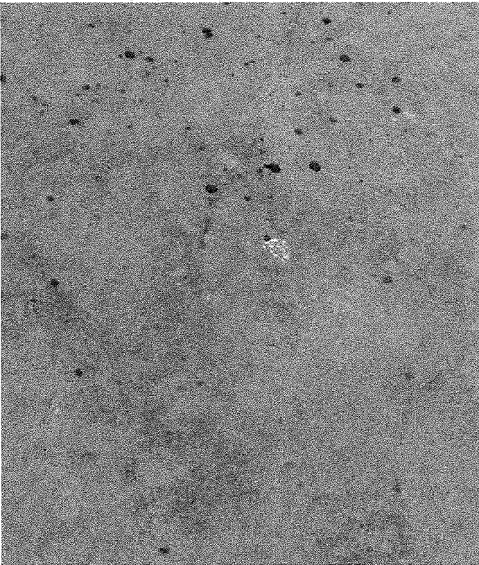
Properly prepared concrete substrate
