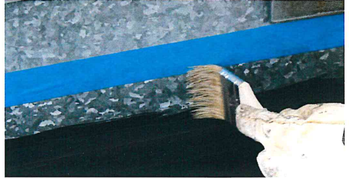
Prime all metal surfaces with M-Prime.
