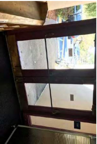
#11 A-B DOOR HARDWARE AGED AND STICKING
