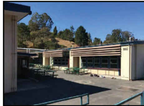
PHOTO - 7 SHADING DEVICES Shading device upgrades would help provide cooling for classrooms without air conditioning
