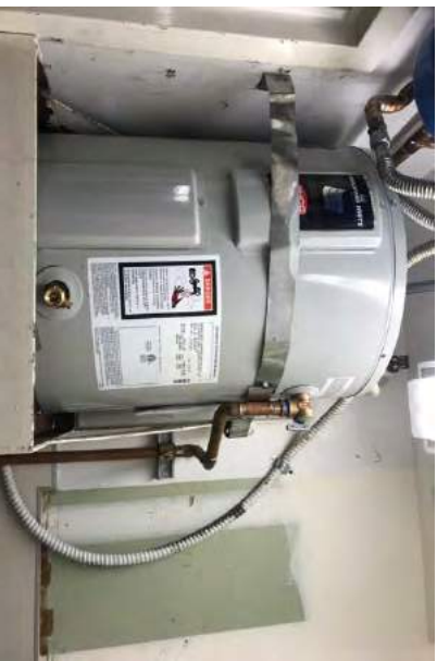
#40 ELECTRIC WATER HEATER
