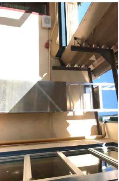
#14 A-B ROOF ACCESS
