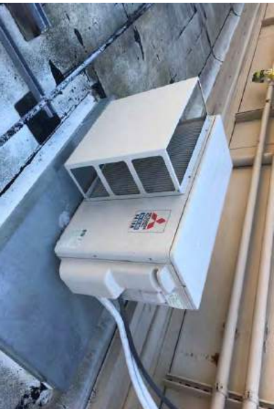
#53 A-B 1.5 TON DUCTLESS SPLIT SYSTEM
