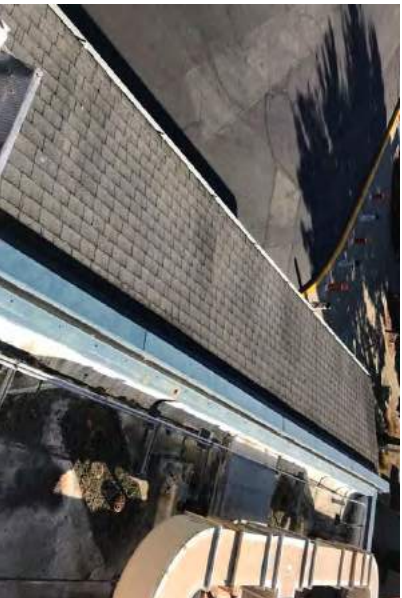
#15 A-B ASPHALT SHINGLE ROOF
