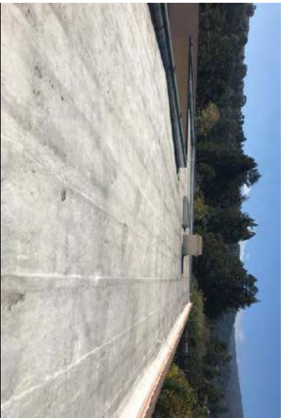
#13 MODIFIED BITUMINOUS ROOF WITH REFLECTIVE COATING
