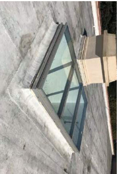
#13 MODIFIED BITUMINOUS ROOF WITH REFLECTIVE COATING
