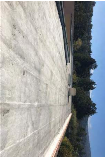
#13 MODIFIED BITUMINOUS ROOF WITH REFLECTIVE COATING
