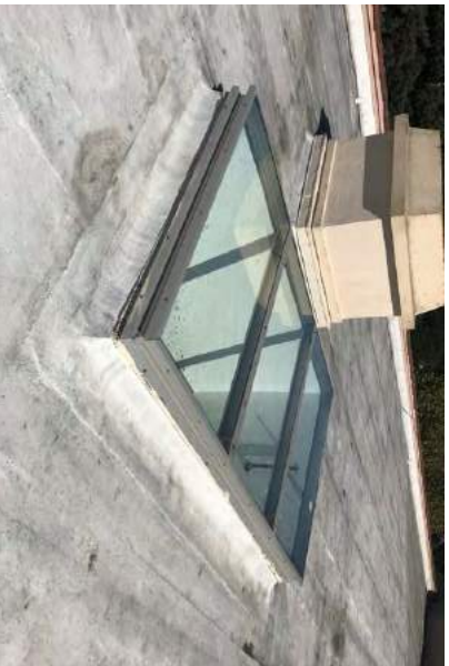
#13 MODIFIED BITUMINOUS ROOF WITH REFLECTIVE COATING
