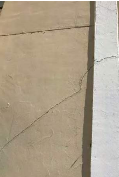
#7 STUCCO CRACKING
