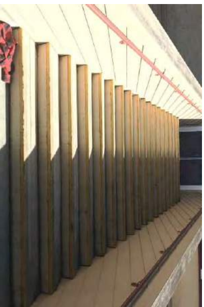
#28 EXTERIOR STAIRS ANNEX BUILDING
