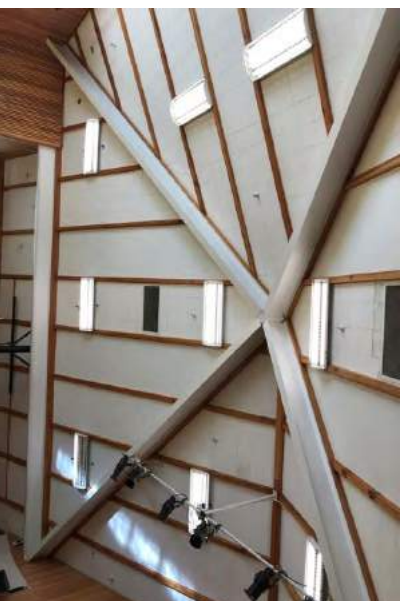
#20 STEEL ROOF BEAMS IN MULTIPURPOSE BUILDING
