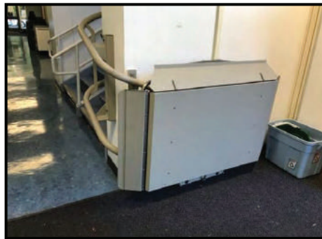
PHOTO - 6 WHEELCHAIR LIFT
