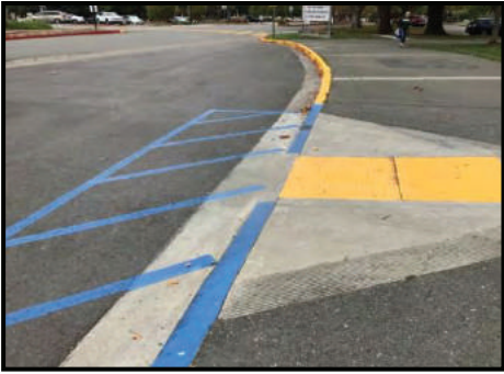
PHOTO - 1 PARKING LOT CURB
