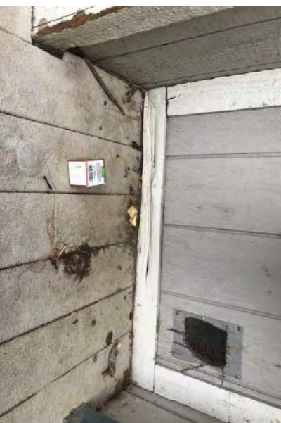
#22 WALL AND DECK AT PORTABLES
