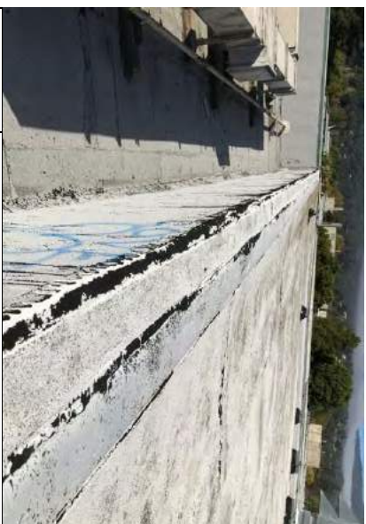
#64 ROOFING DETERIORATION
