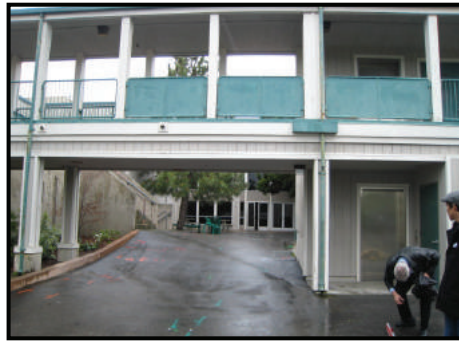
PHOTO - 2 MAIN BUILDING EXTERIOR
