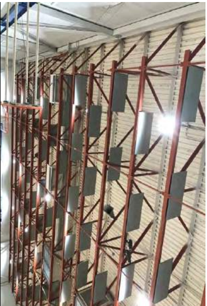
#19 CEILING OF GYM
