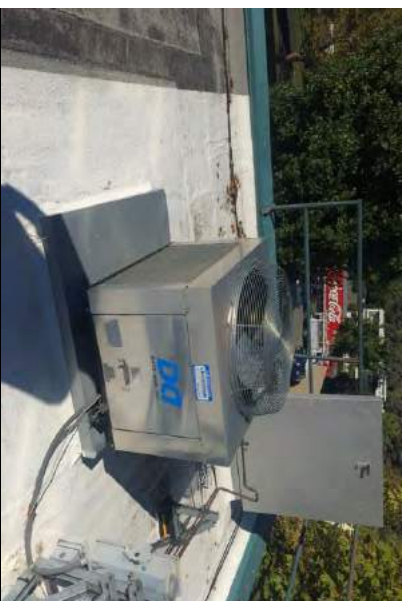
#44 DRYCOOLER/CONDENSER, AIR-COOLED
