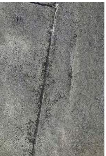
#6 ROOF, MAIN BUILDING
