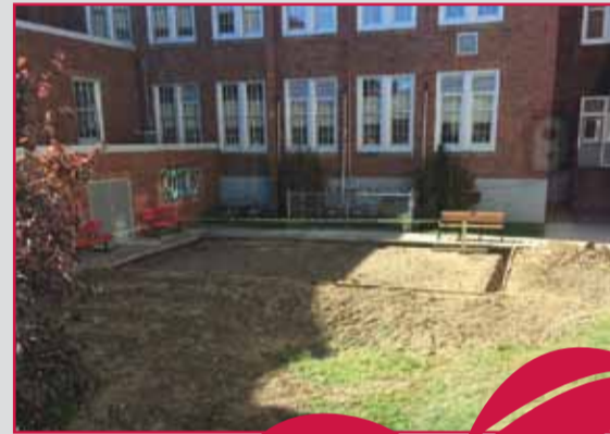
The first stages on the layout of the greenhouse in November.
