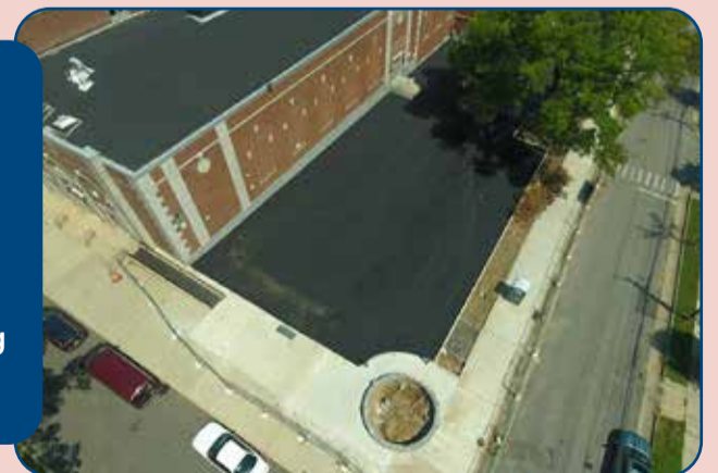
New asphalt, lighting, concrete and fencing were all added during the Middle School's parking lot construction.
