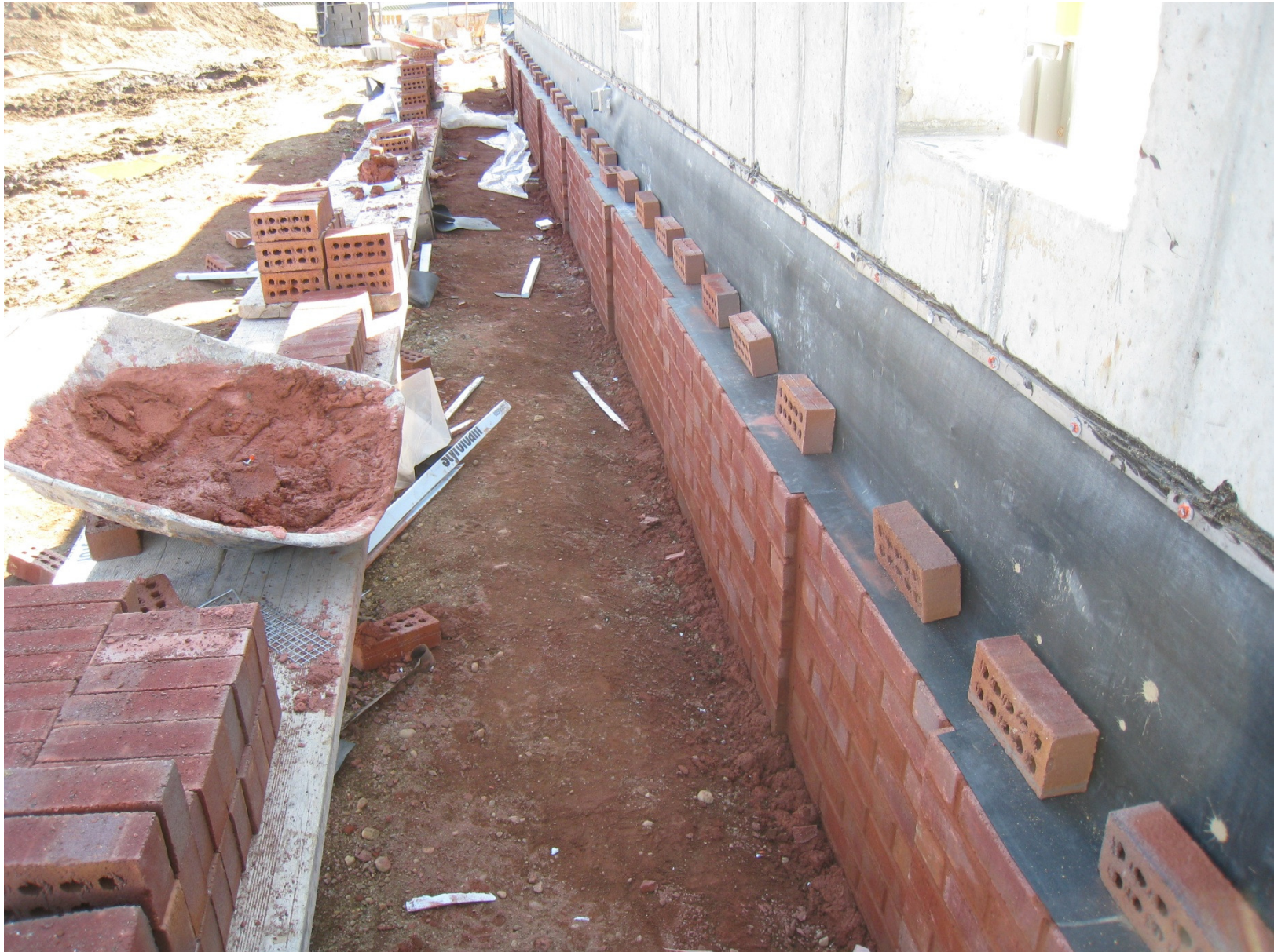
Starting the brick work (February 2012)
