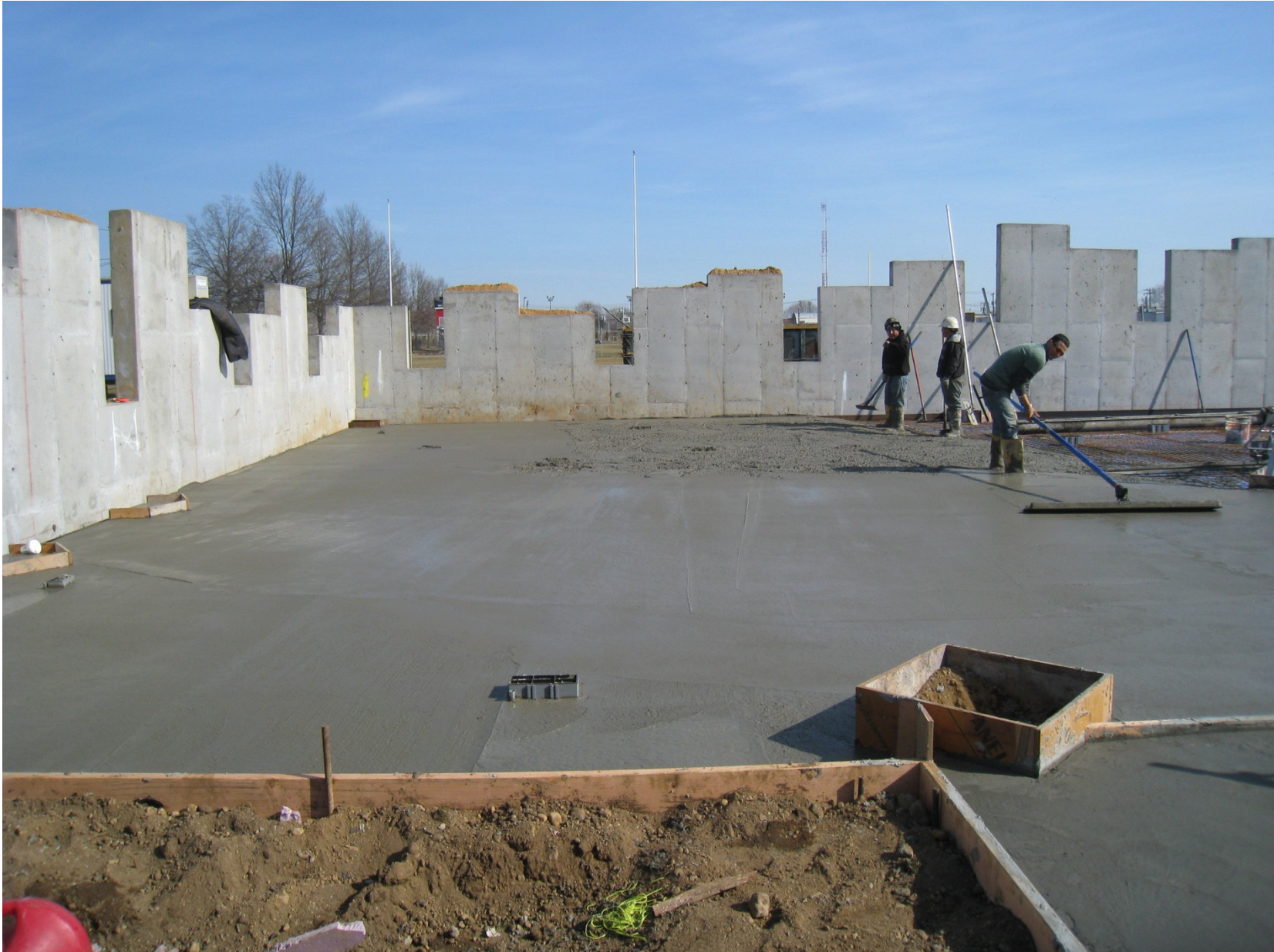
Concrete floor slabs (February 2012)
