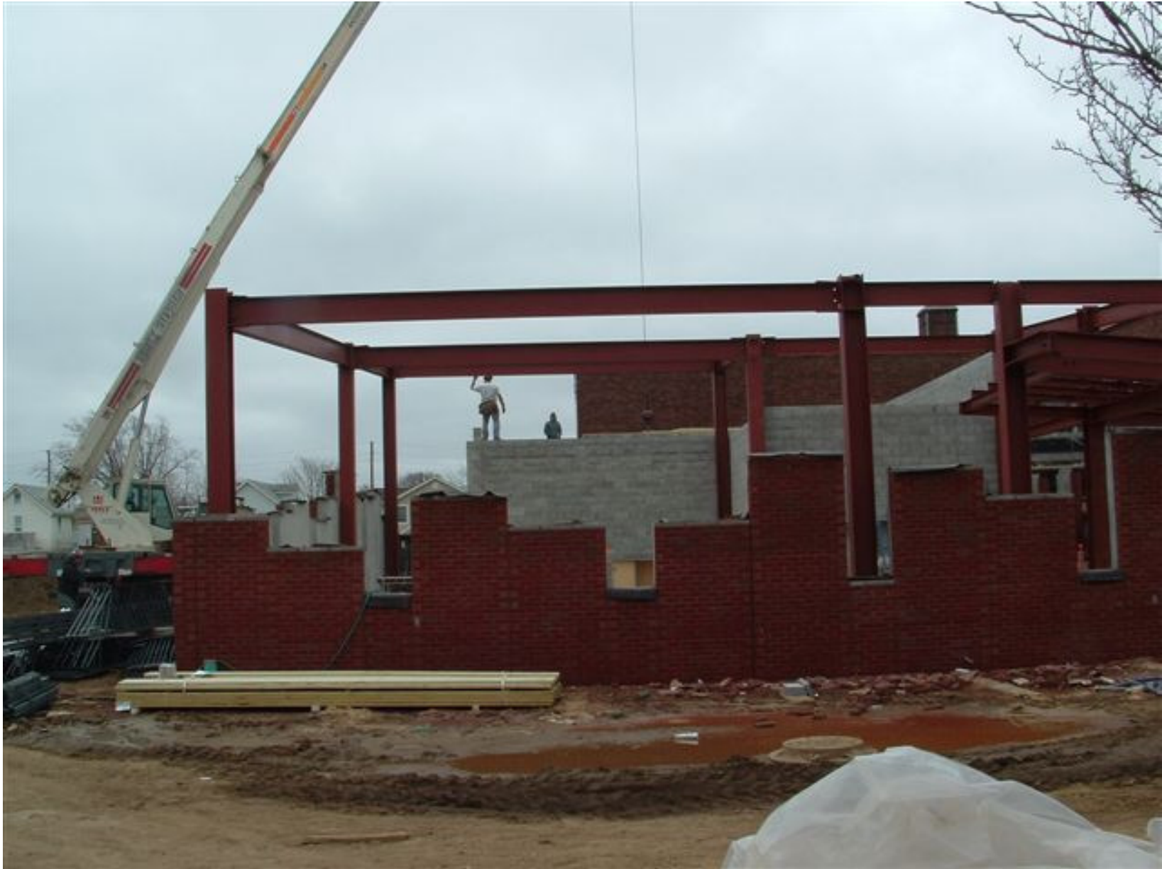
First day of the steel erection (March 2012)
