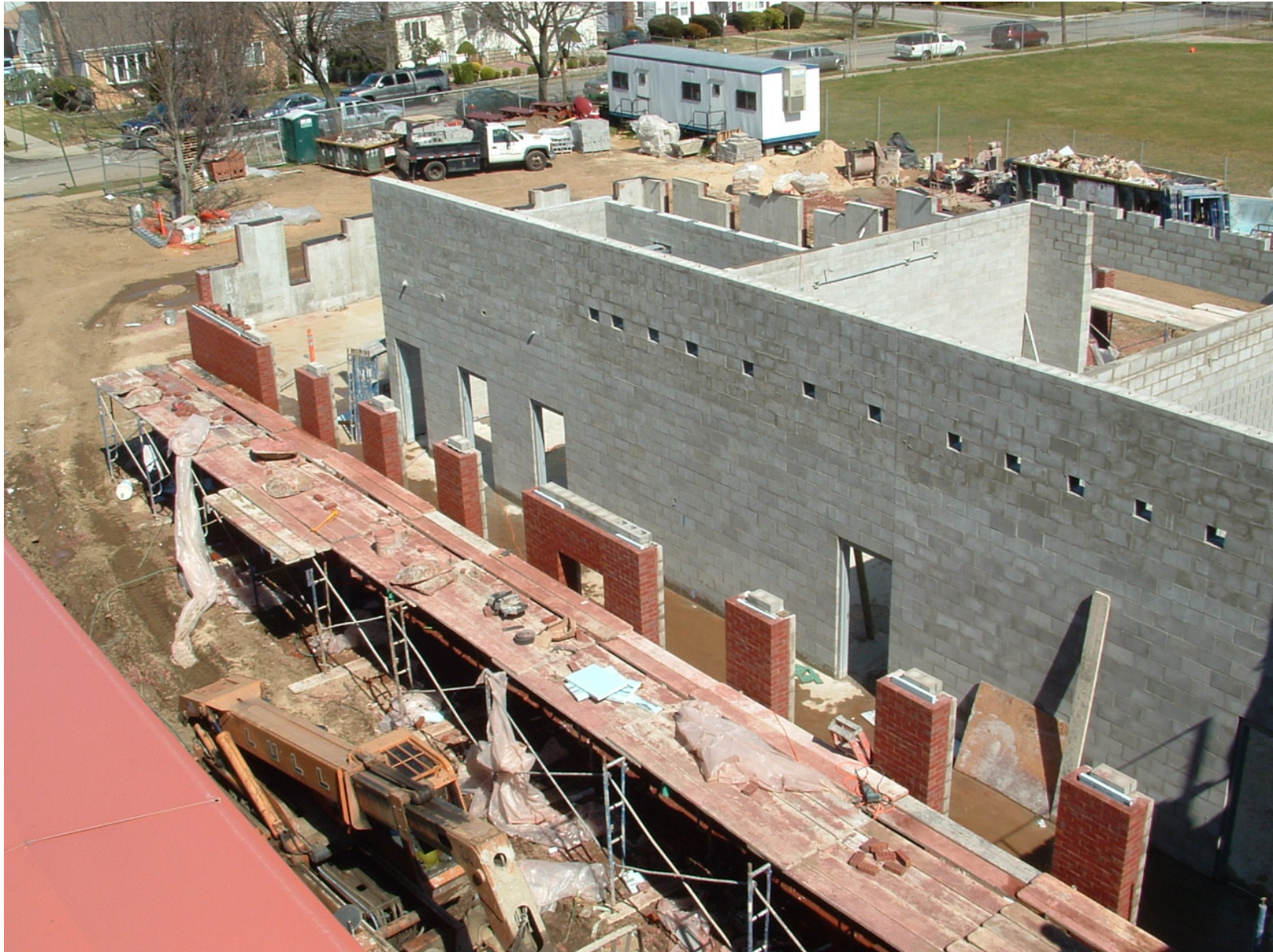
Progress with the brick work (March 2012)
