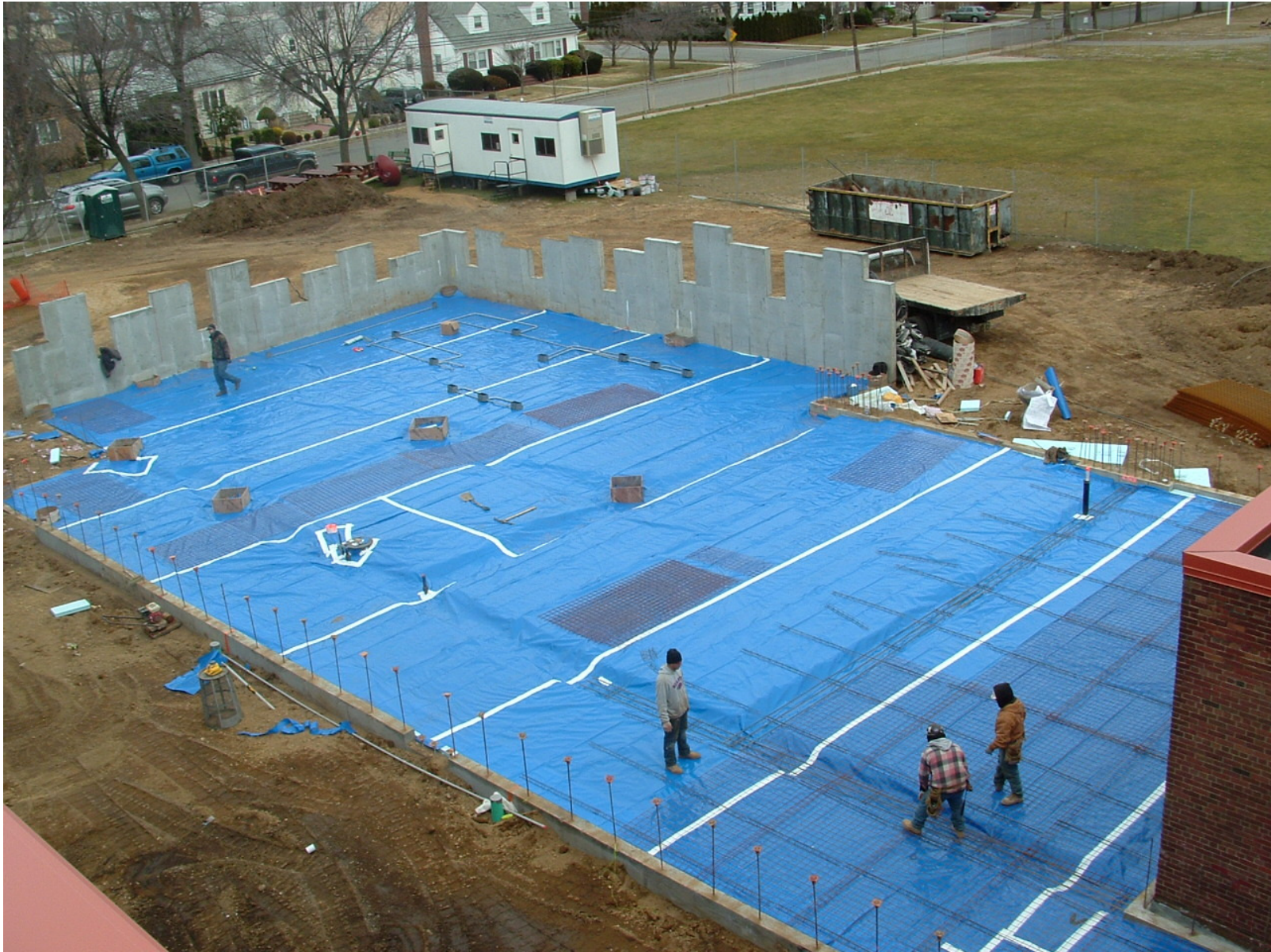
Progress with concrete walls and slabs (February 2012)
