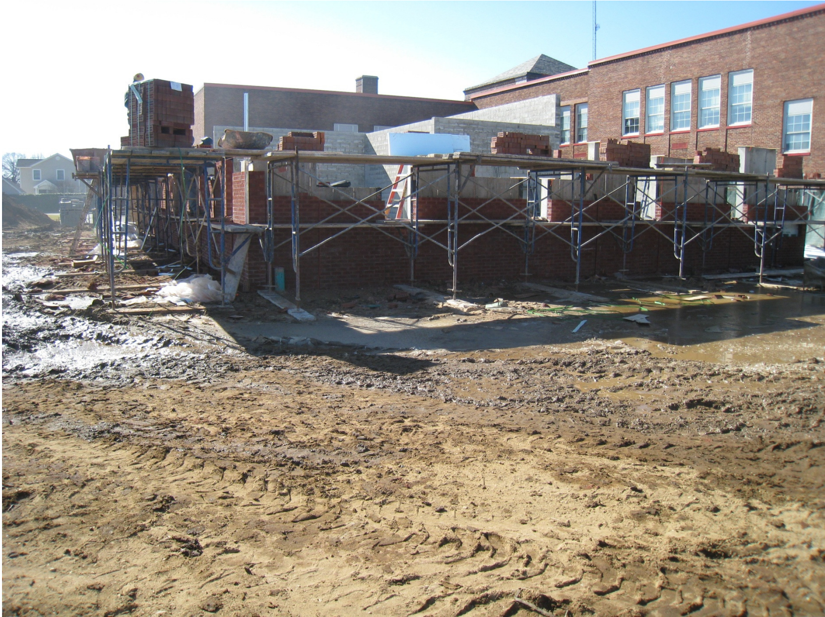
Progress with the brick work (February 2012)
