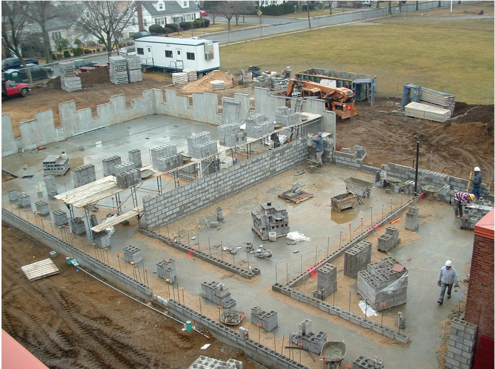
Masonry bearing walls (February 2012)
