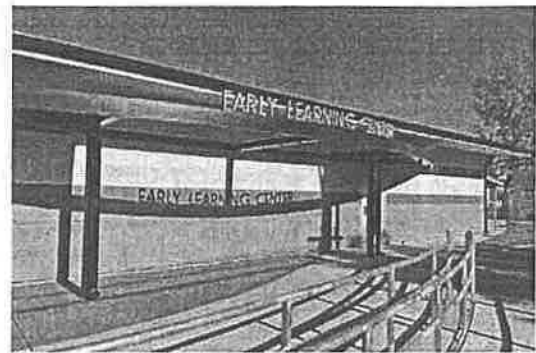
Jordan ES: Portables to Permanent, Sewer, Roofing, HVAC, Fire Alarm
