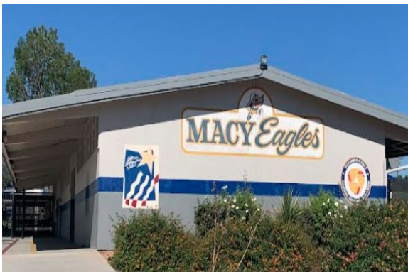
Macy ES: Roofing, HVAC, Fire Alarm, Sewer, Storm Drain
