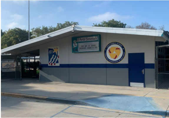
El Portal ES: Roofing and Fire Alarm
