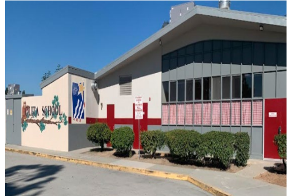
Olita ES: Roofing, HVAC, and Fire Alarm
