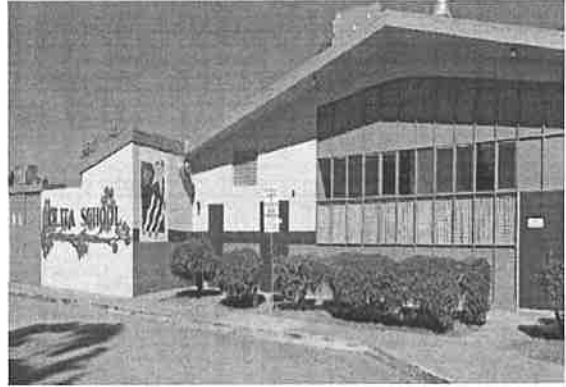
Olita ES: Roofing, HVAC, and Fire Alarm
