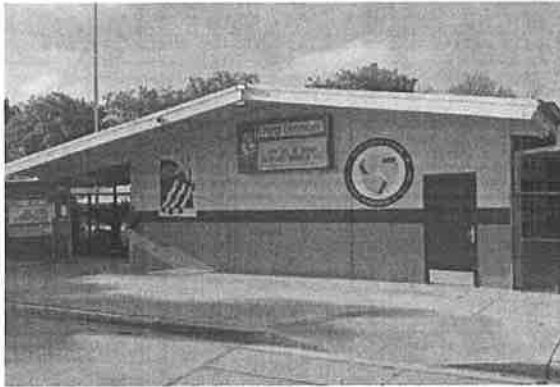
El Portal ES: Roofing and Fire Alarm
