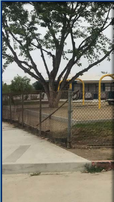
Macy Kindergarten Security Fence - Before
