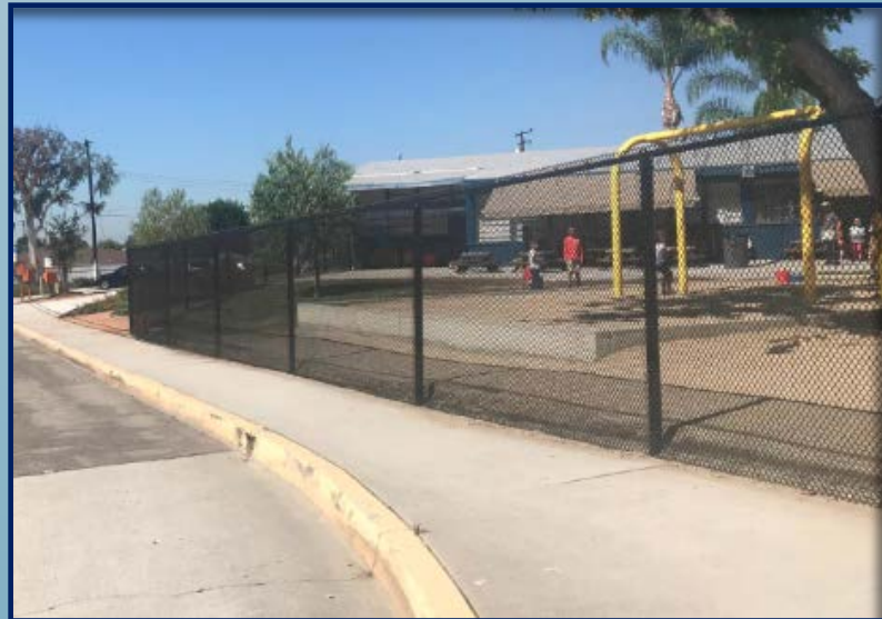
Macy Kindergarten Security Fence - After
