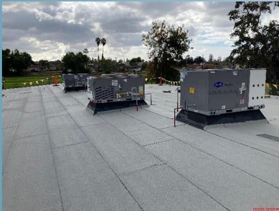
Roofing and Units
