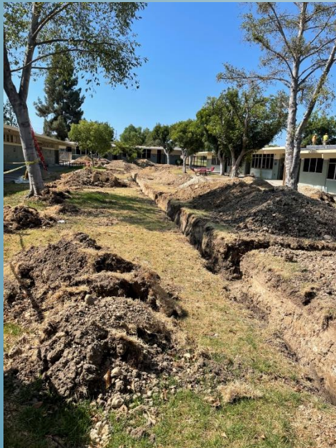
Storm Drain & Electrical
