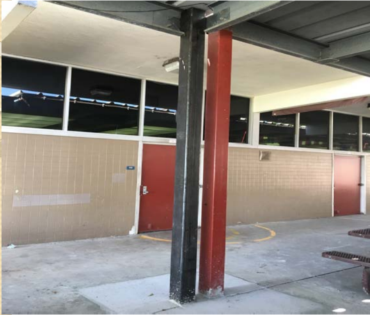
New Column Completed
