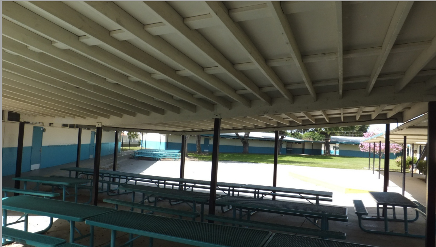
E-2: SITE REQUESTED INSTALLATION OF SHADE SHELTER IN QUAD.
