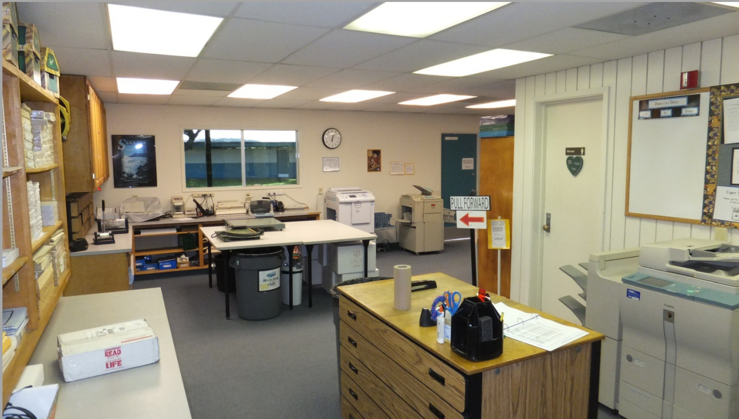
E-3: ADMINISTRATION BUILDING ADDITION REQUIRES CORRECTIVE ACTION TO COMPLY WITH CURRENT CODES
