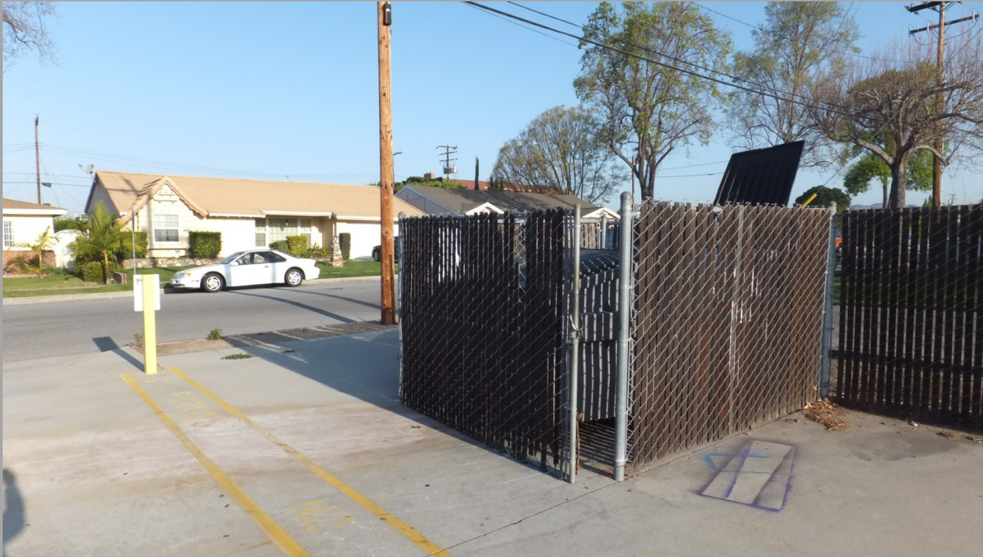
J-1: TRASH ENCLOSURE IN PARKING LOT NOT LOCATED CONVENIENT TO AREAS OF GREATEST CONCENTRATION OF TRASH.
