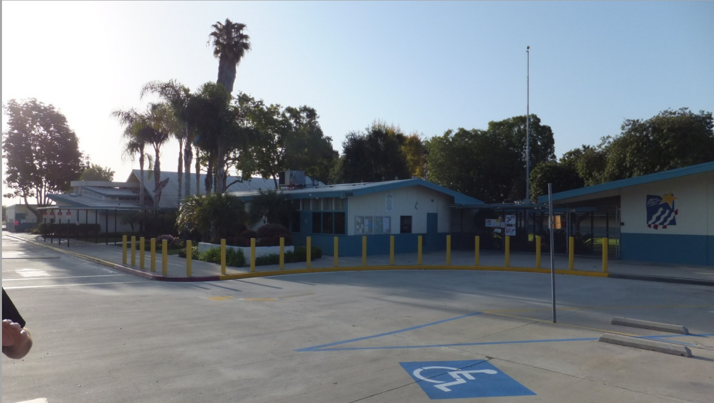
D-11: STUDENT DROP-OFF AREA NEEDS IMPROVEMENT. SCHOOL REPORTS LONG DELAYS AND TRAFFIC PROBLEMS RELATED TO STUDENT DROP-OFF AND PICK-UP.
