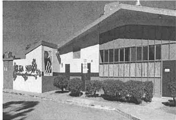
Olita ES: Roofing, HVAC, and Fire Alarm
