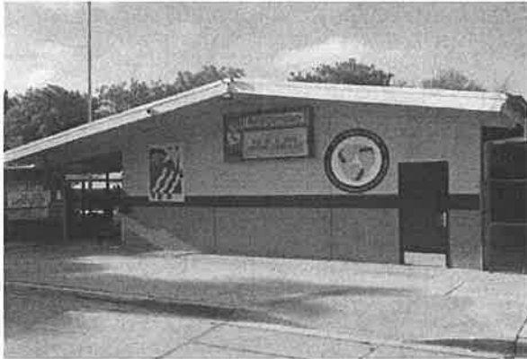
El Portal ES: Roofing and Fire Alarm
