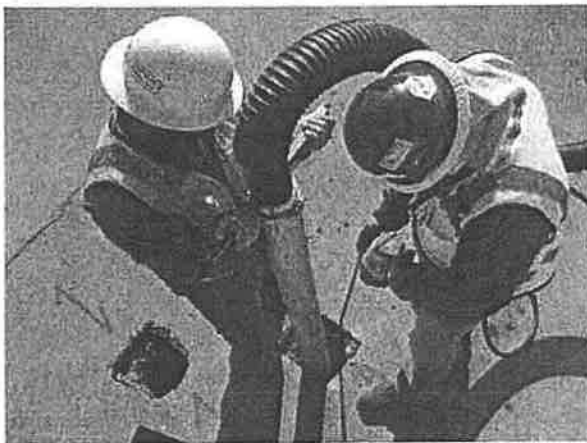
C Below technicians performing potholing
