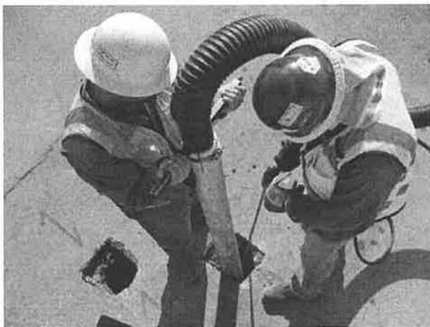
C Below technicians performing potholing
