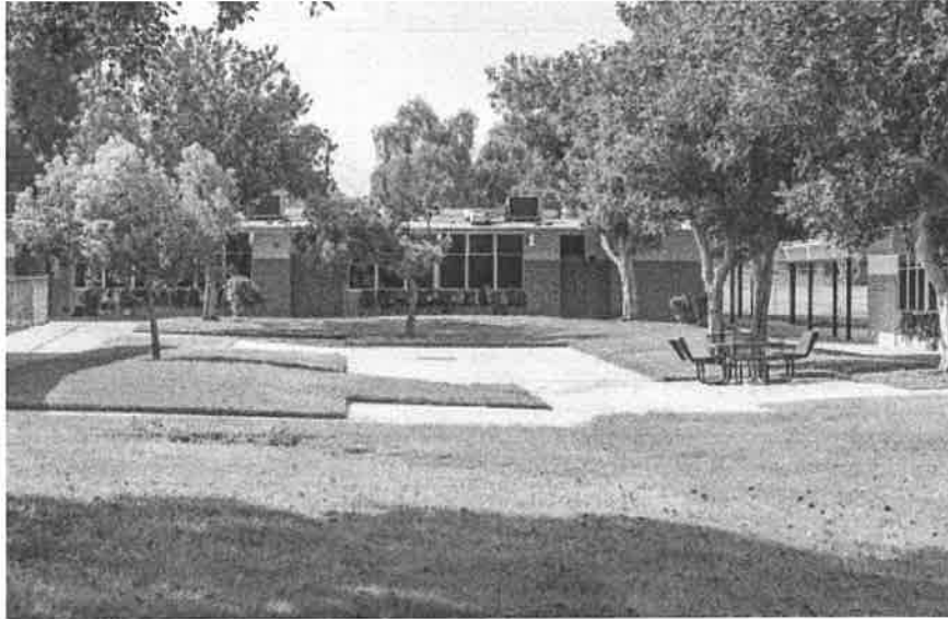
Meadow Green ES: Roofing, HVAC, Fire Alarm, Sewer
