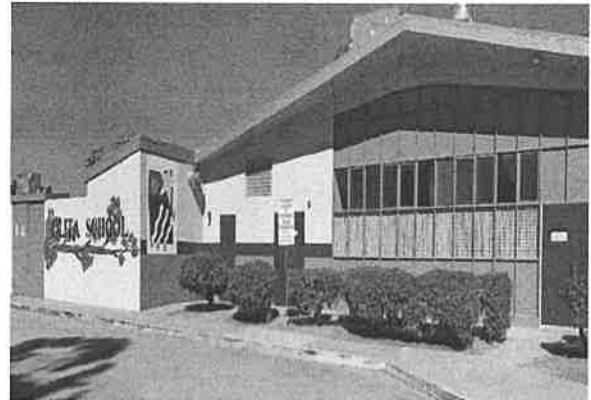
Olita ES: Roofing, HVAC, and Fire Alarm
