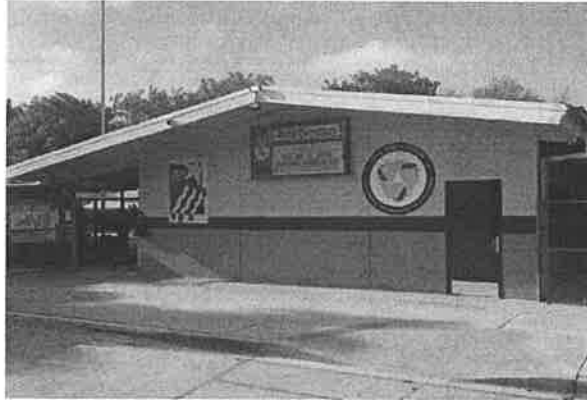
El Portal ES: Roofing and Fire Alarm
