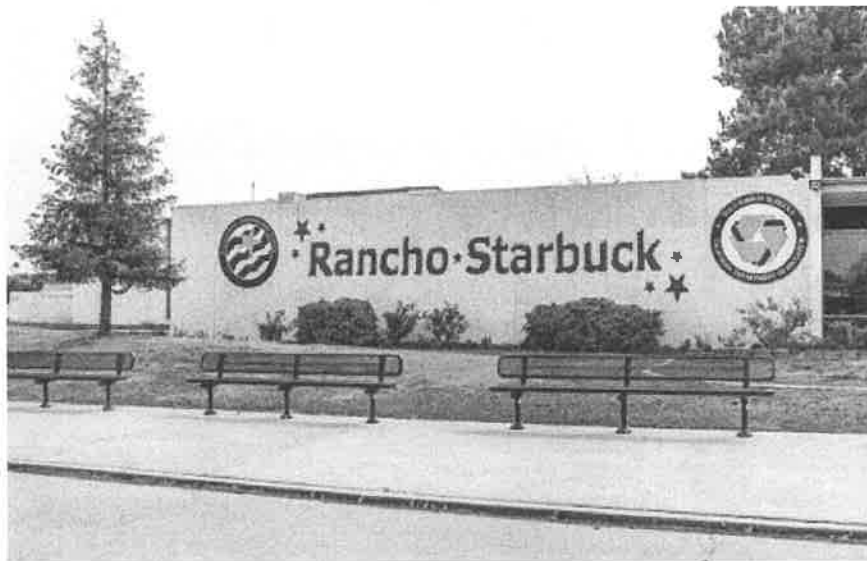
Rancho Starbuck IS: Roofing, HVAC, Fire Alarm, Sewer
