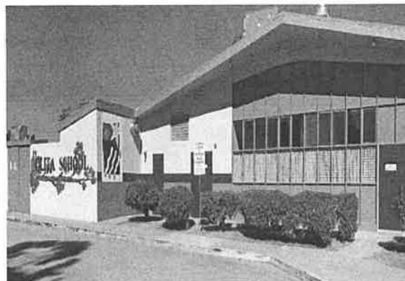
Olita ES: Roofing, HVAC, and Fire Alarm
