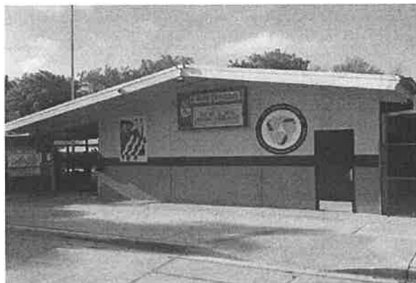
El Portal ES: Roofing and Fire Alarm
