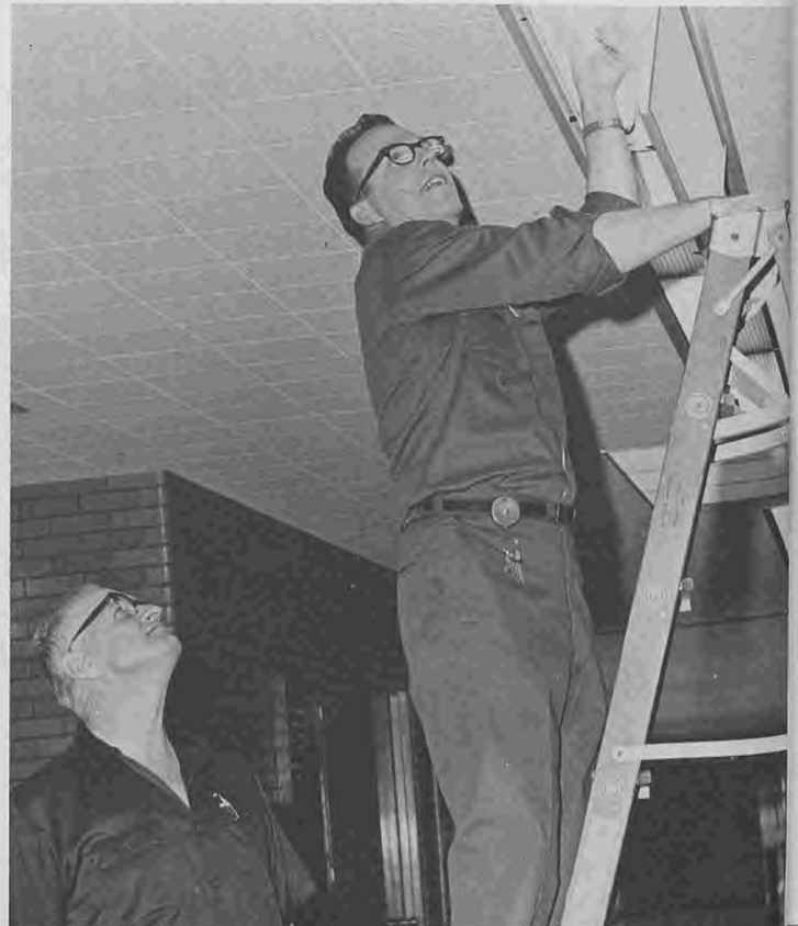
Performing one of their assignments as custodians, Orvid Pitcher installs a new fluorescent light fixture while Angus Esplin supervises the job.
