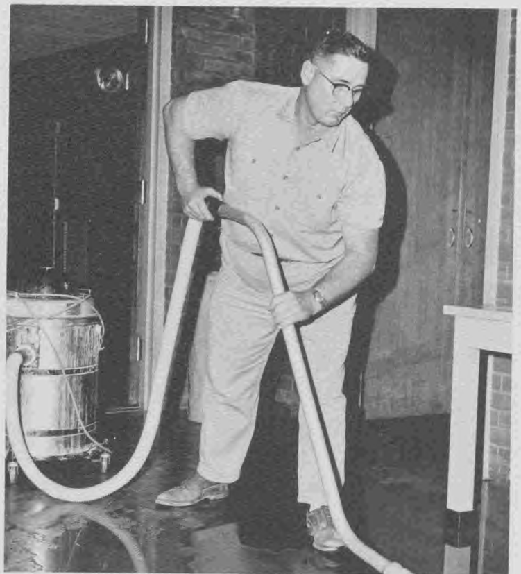
Mr. Ed Hyden vacuums the water that leaked through the ceiling of the biology room following the first snow storm.
