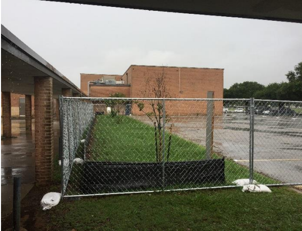
Lamar CHS Construction Fencing
