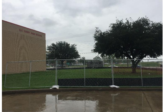
Terry HS Construction Fencing
