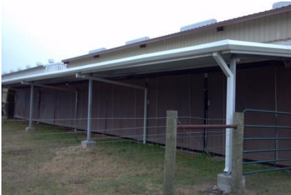
Ag Barn renovations
