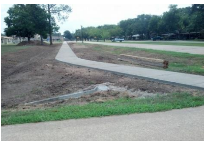
Bowie Elementary School
