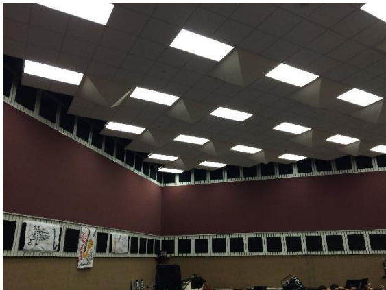
Terry High School Band Hall Addition
