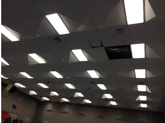
Lamar Consolidated High School Band Hall Addition
