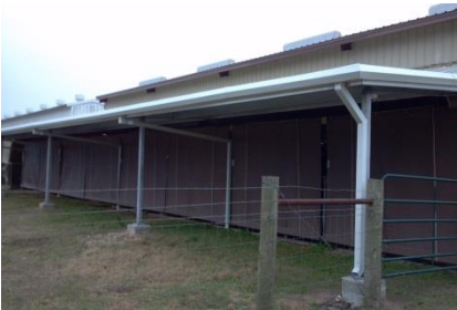
Ag Barn renovations
