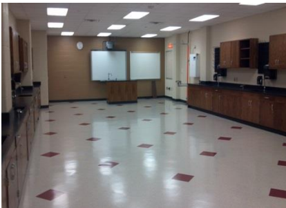
George Ranch HS Shell Build-Out
