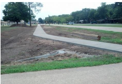
Bowie Elementary School
