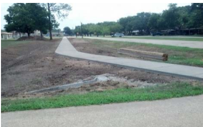
Bowie Elementary School
