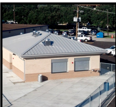
Traylor Stadium Renovations
