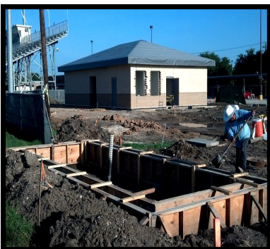
Traylor Stadium Renovations
