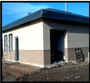
Traylor Stadium Renovations
