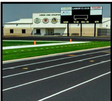
Traylor Stadium Renovations
