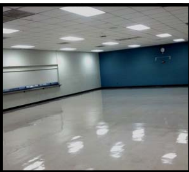
Miscellaneous Renovations / Jackson ES
