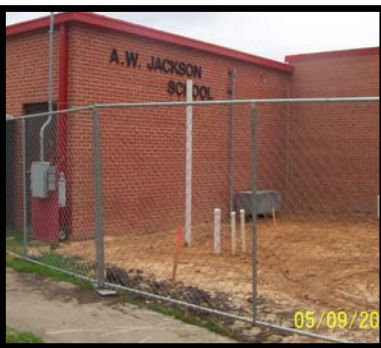
Miscellaneous Renovations / Jackson
