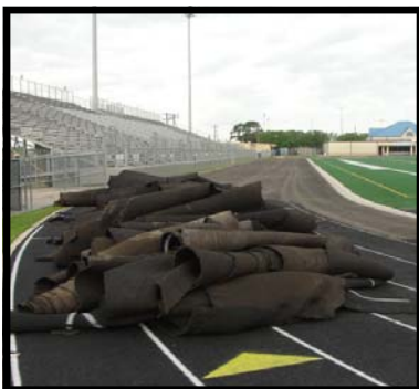
Traylor Stadium Renovations
