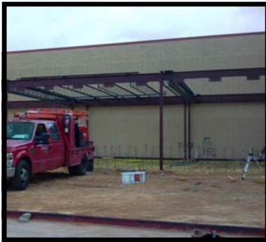
Miscellaneous Renovations / Terry HS
