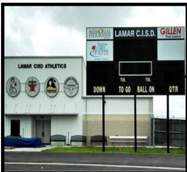
Traylor Stadium Renovations
