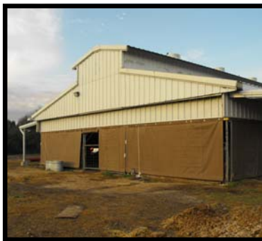
Agricultural Barn Renovations
