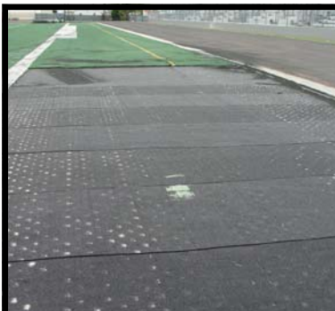
Traylor Stadium Track & Turf
