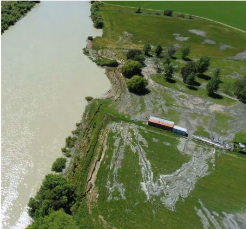
Figure 4.68: Aerial view of liquefaction manifestation at the Blenheim Rowing Club looking east (18 Nov 2016, approx. centre of image: S41.4883, E174.0096, Marlborough Regional Council, 2016).
