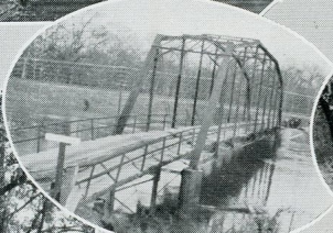
Wint Creek Bridge
