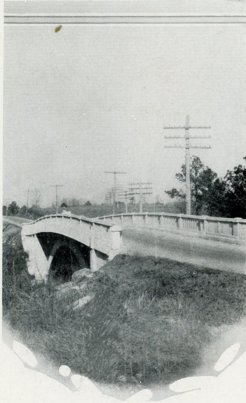
"Shoal Creek Bridge"
